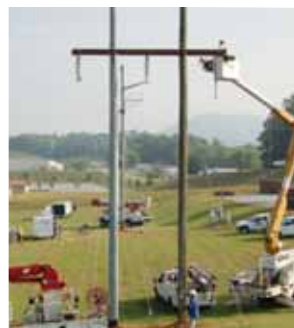
Linemen receive training on transmission line construction and repair.
